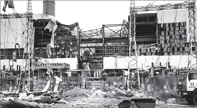
Zmiivska TPP after Rashist shelling. Photo: Open source
