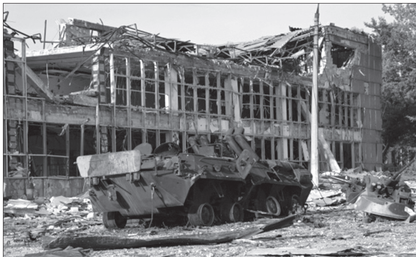
Destroyed Mariupol Ilyich Iron and Steel Works. Photo: Open source
